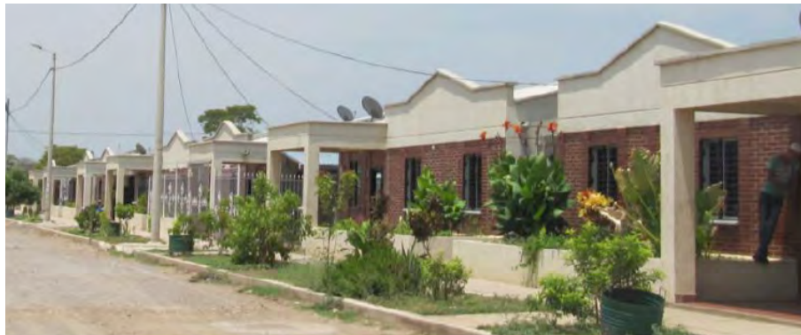
Figure 6. A street in the new settlement site of Roche
