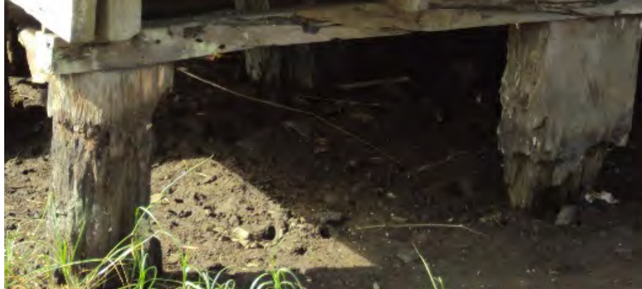
Figure 6. Weathered of wood of the stilts houses
