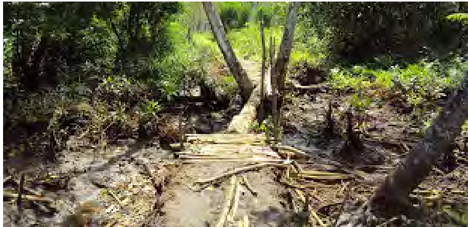
Figure 7. Repeatedly destroyed makeshift walkway
