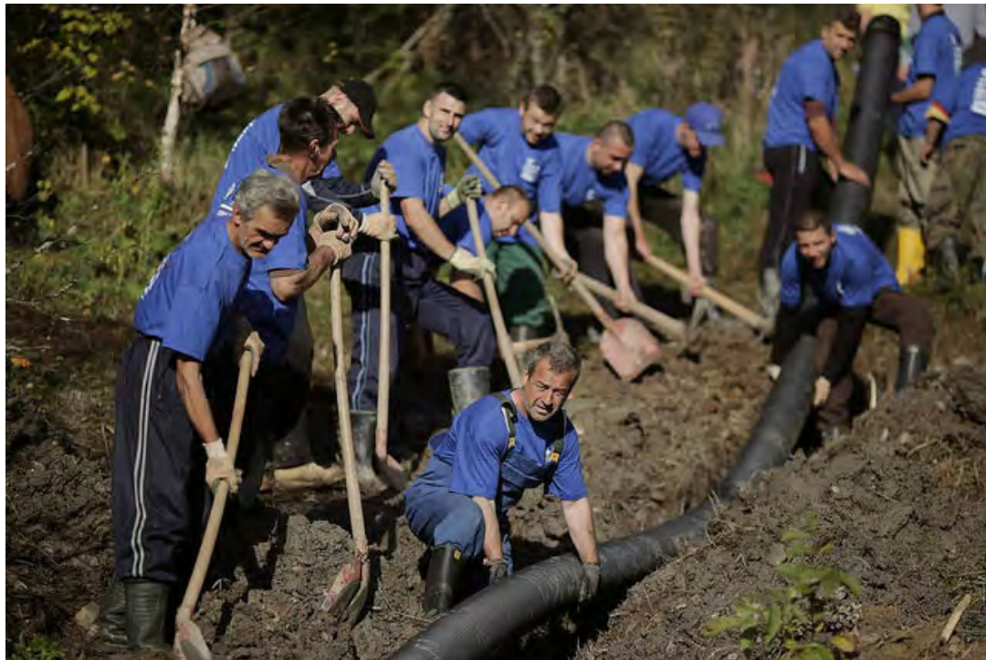
Photo 5. Landslide rehabilitation in Vares by the “Cash for Work” programme.
