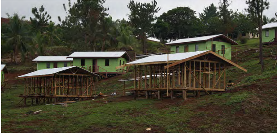
Figure 11. Houses under construction in April 2013
