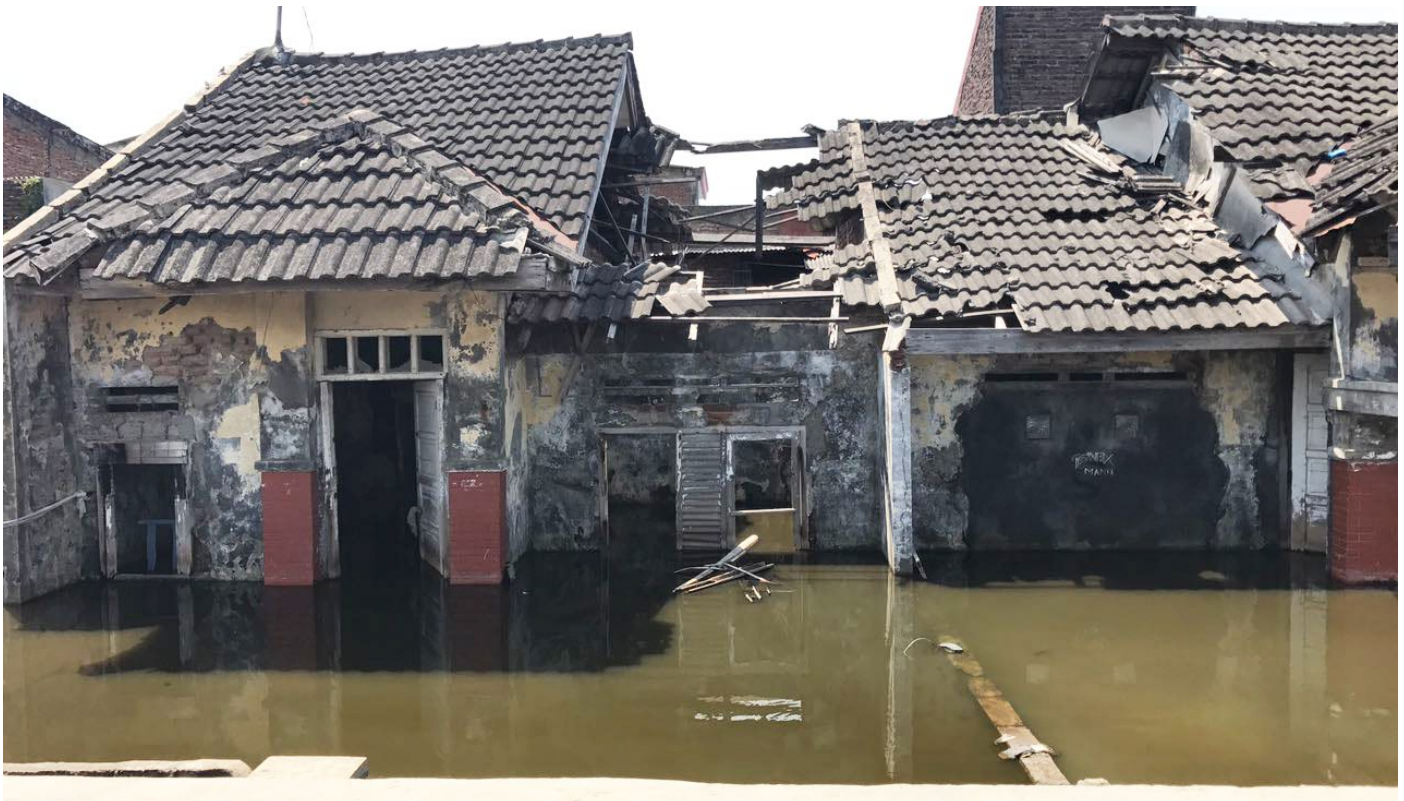
Houses affected by land subsidence on the outskirts of Semarang. © Adriana SIERRA LEAL and Meylin GONZALES HUAMAN 2017
