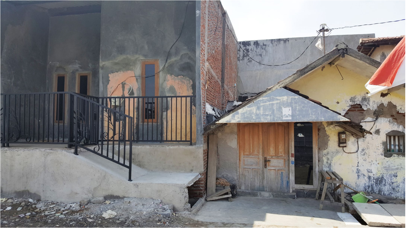
Houses affected by land subsidence in Demak. The ground floor of the house on the left has been elevated as a response to subsidence and rob . © Adriana SIERRA LEAL and Meylin GONZALES HUAMAN 2017
