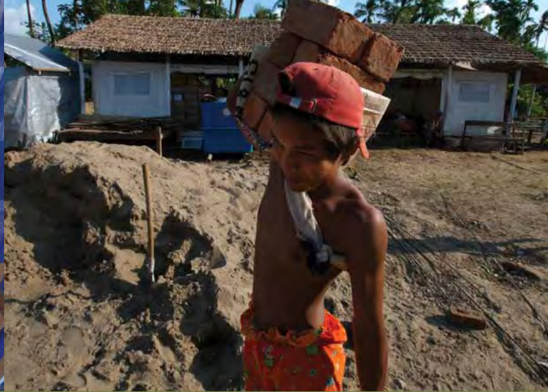
▲ Builders start work on a permanent rural health centre next to the KCCP tent clinic. © IOM 2008 - MMM0346 (Photo: Piers Benatar)
