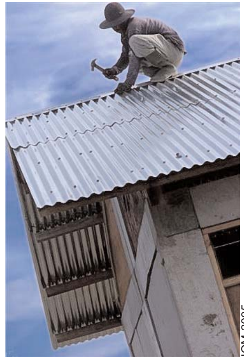
Construction of transitional housing in Banda Aceh.
