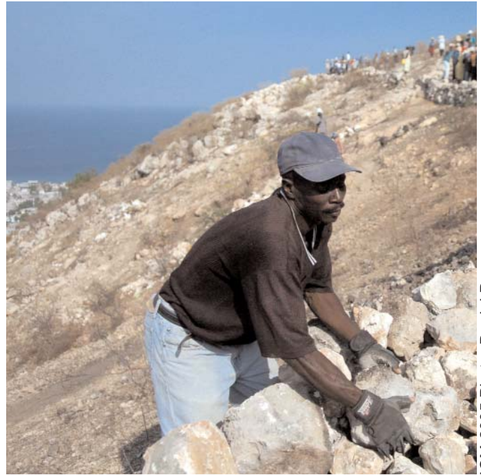
Moving rocks to form a retaining wall.
