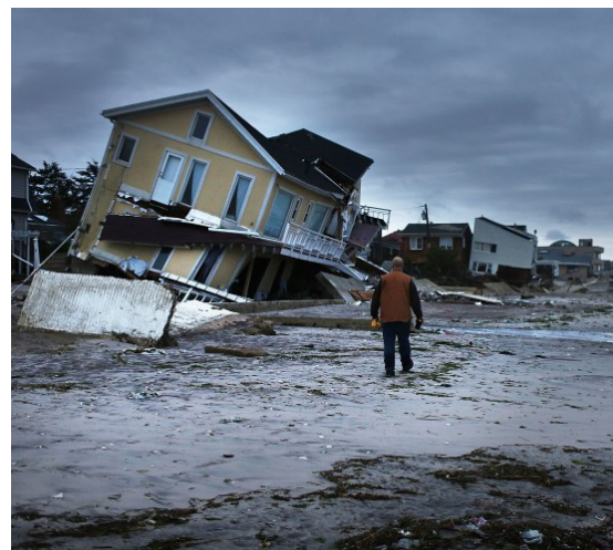
Picture 1. After hurricane Sandy
