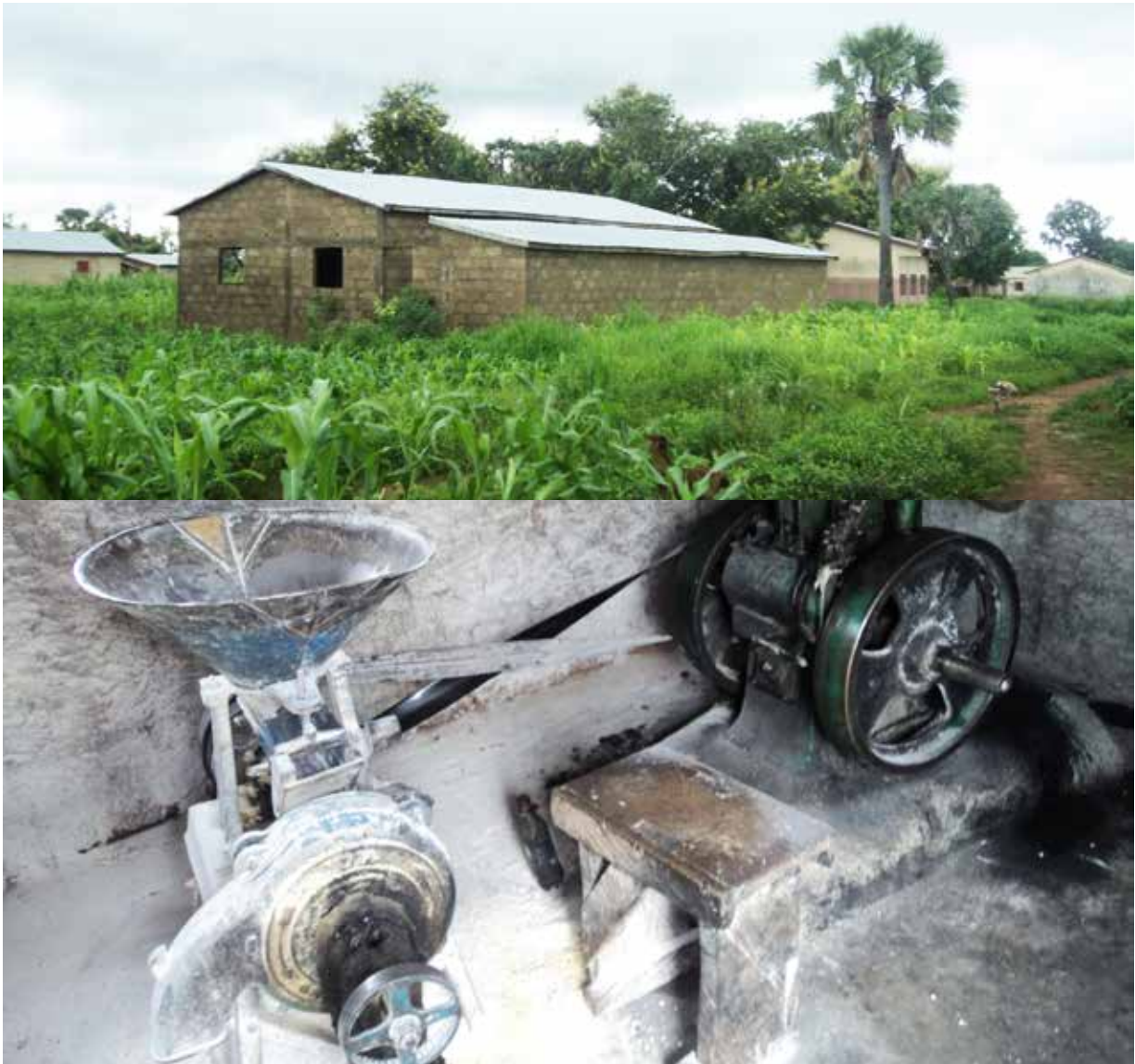
Construction of building and grinding mill with cash remittances (Dassari; Porga) © Vanessa Drier, 2014
