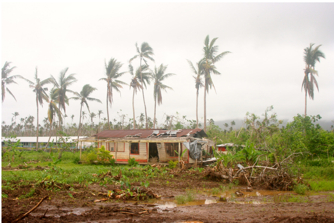
Damages from the 2012 cyclone Evan, Tafitoala village, Samoa. © Loic Le De, January 2013
