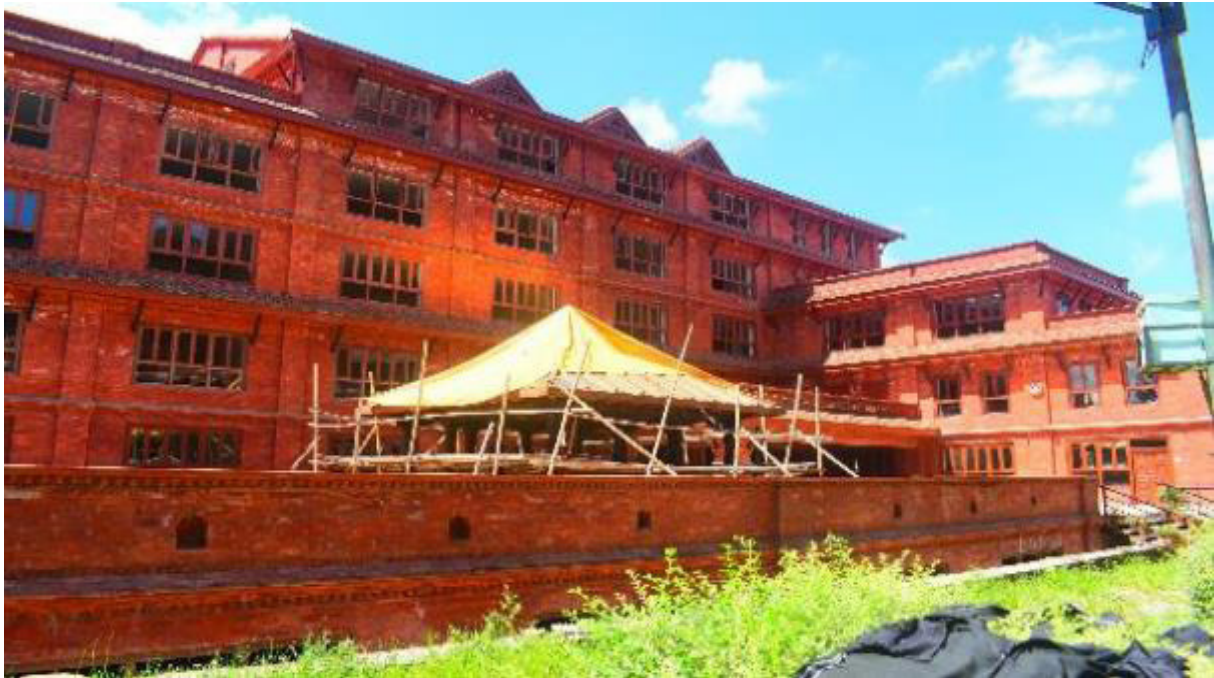
Figure 68. Waiting area built in Khwopa Engineering College's premises
