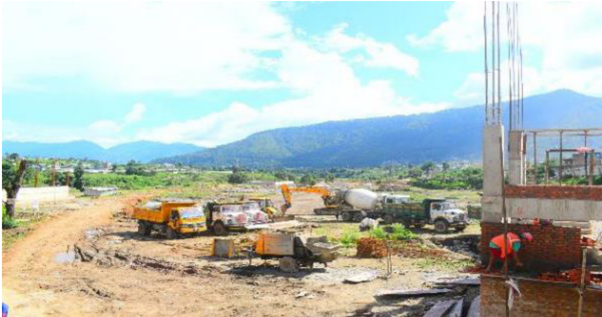
Figure 60. Ongoing construction work for a dry port in Himal Cement Company
