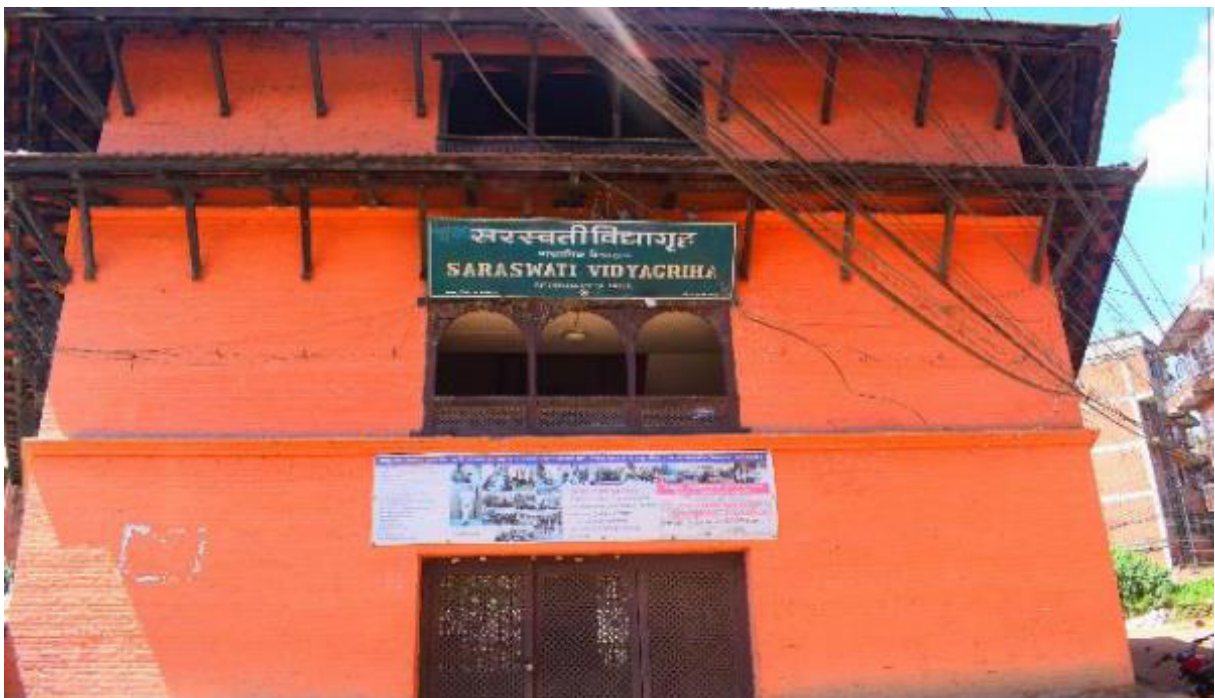
Figure I35. Saraswati Vidyagriha building
