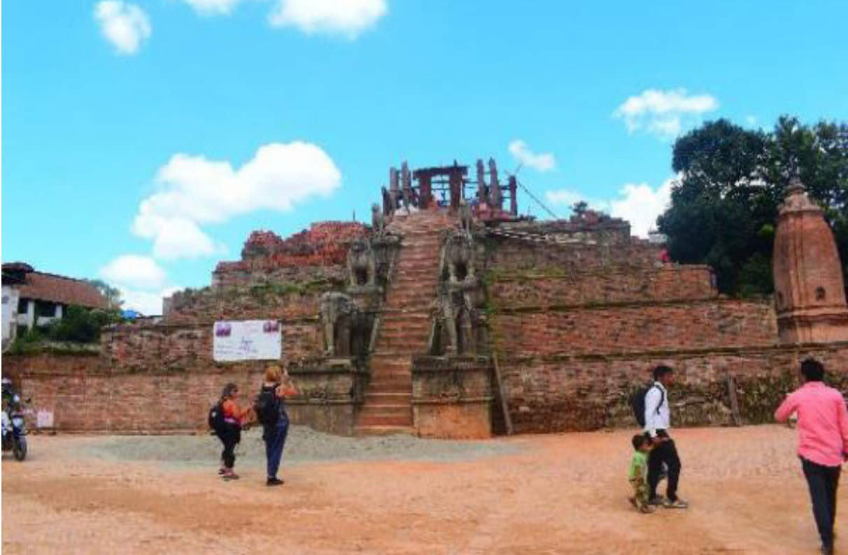
Figure 36. Temple under reconstruction in Bhaktapur Durbar Square
