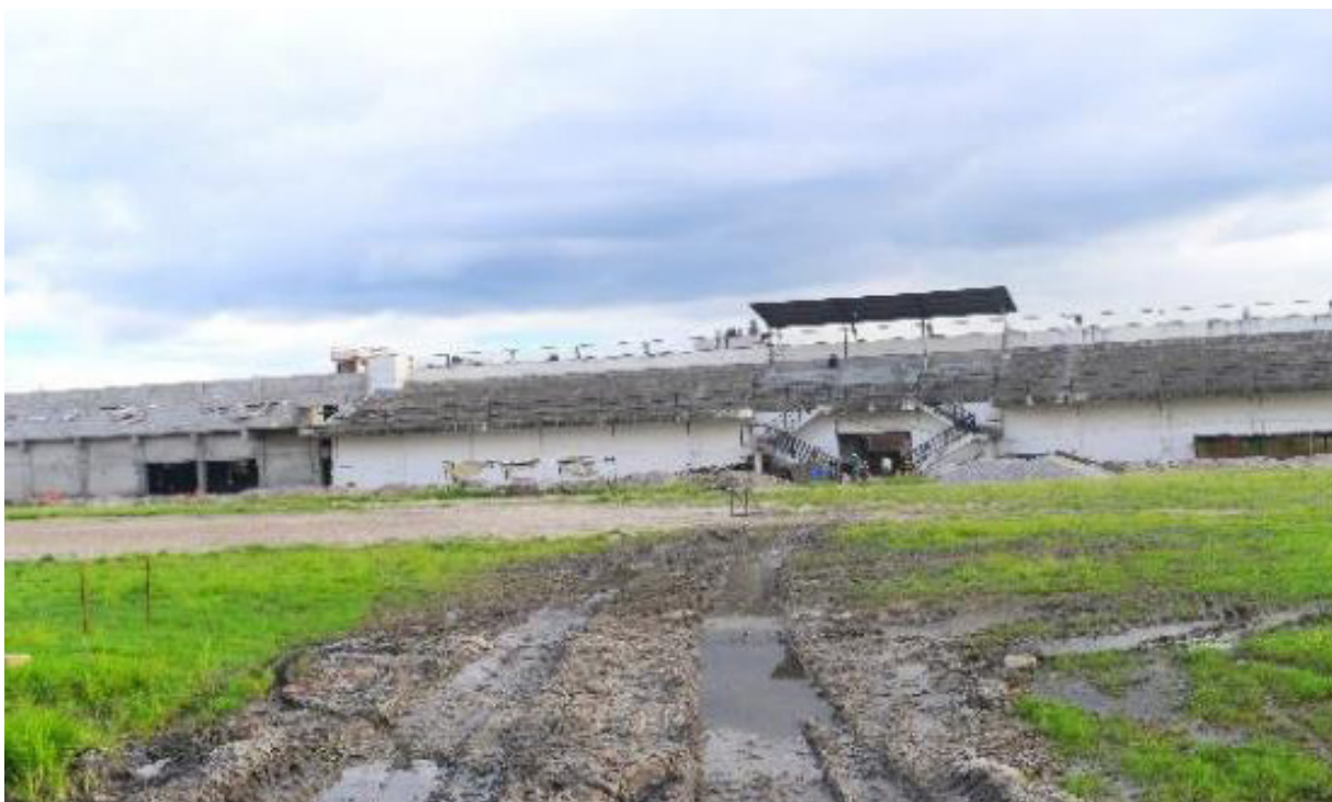
Figure 9. Extension of existing bleachers of ANFA ground
