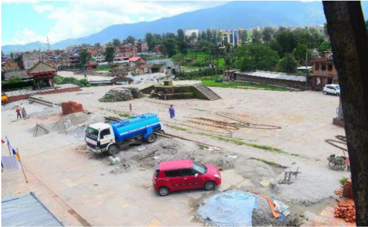
Figure 40. Construction materials accumulated in the open space of Bhelukhel
