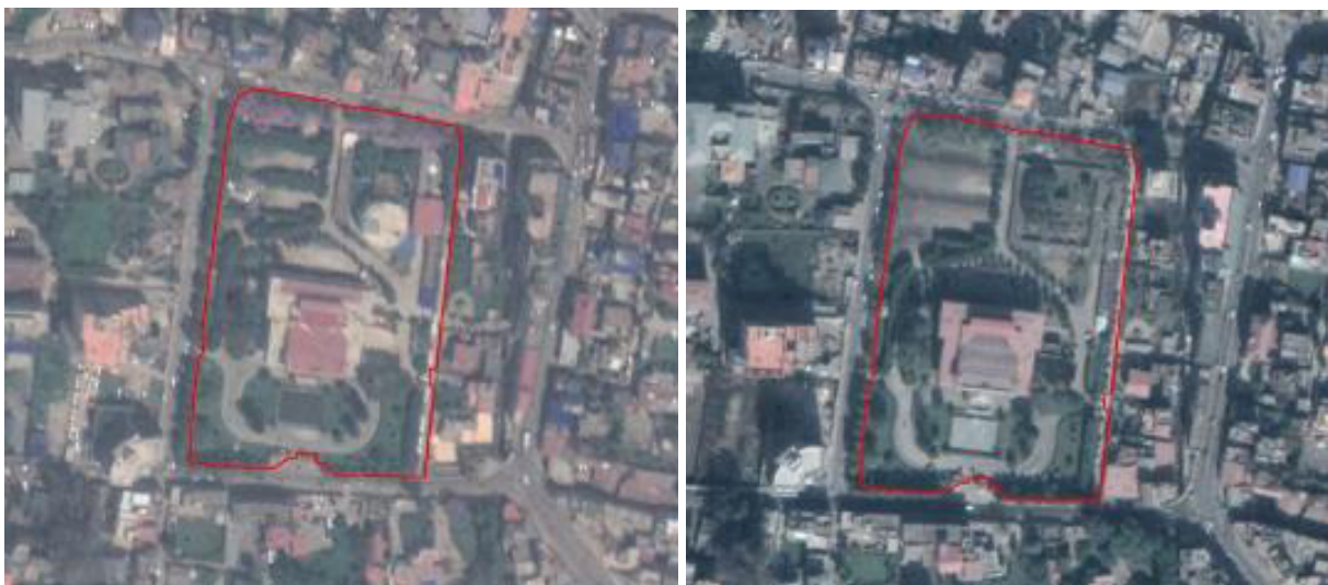
Figure 91. Aerial view of the Nepal Academy in 2013 and 2019
