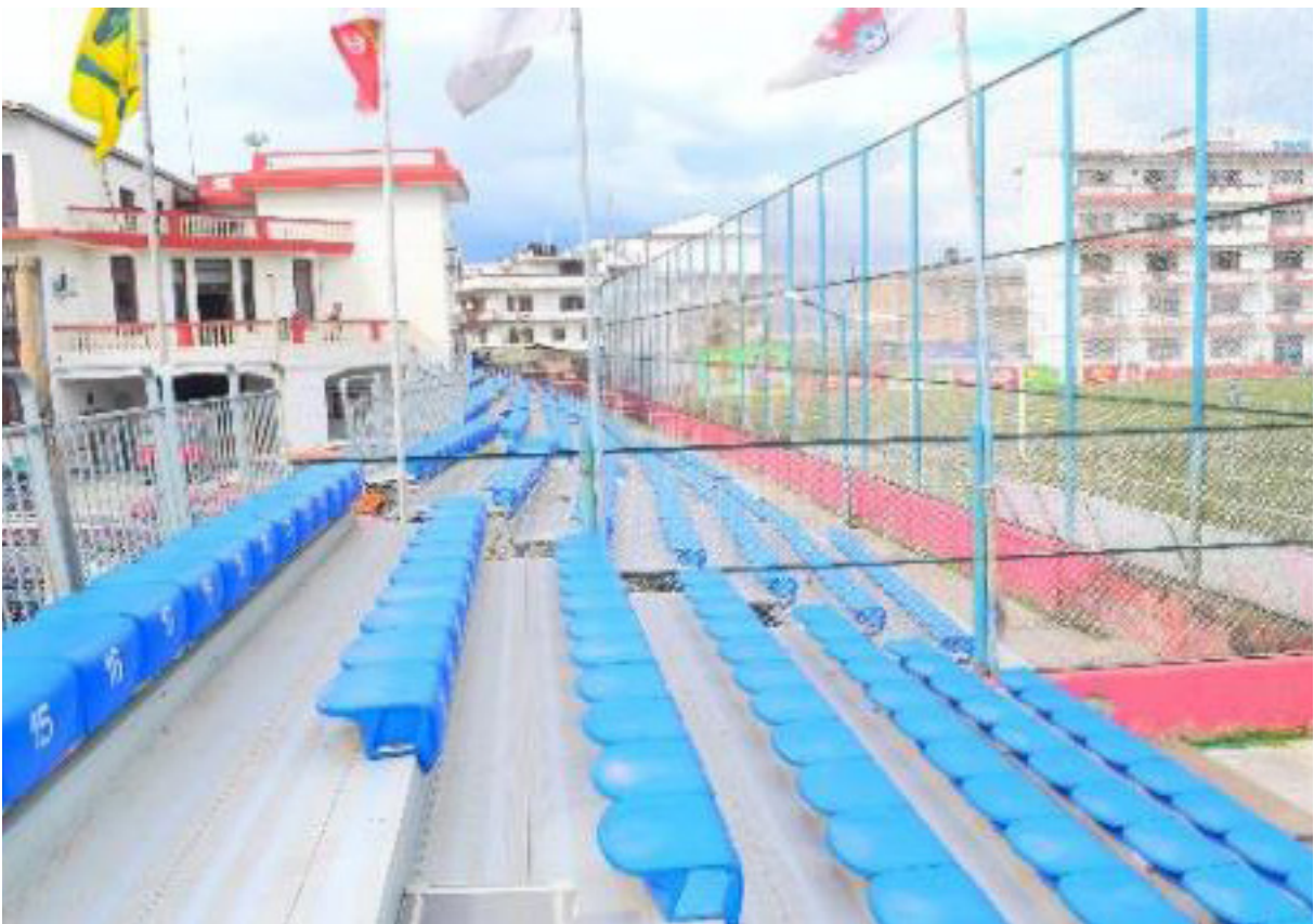
Figure 13. Newly constructed bleachers at ANFA Football stadium
