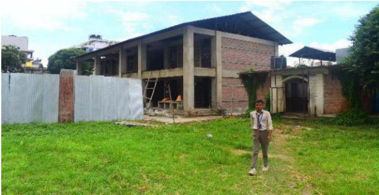
Figure 78. Building under construction in the Madan Smarak school premises
