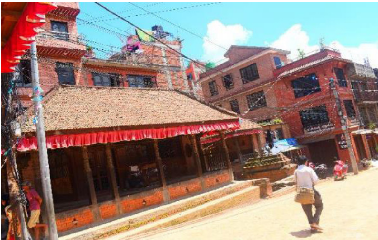
Figure I47. A newly constructed waiting area in Suryamadi
