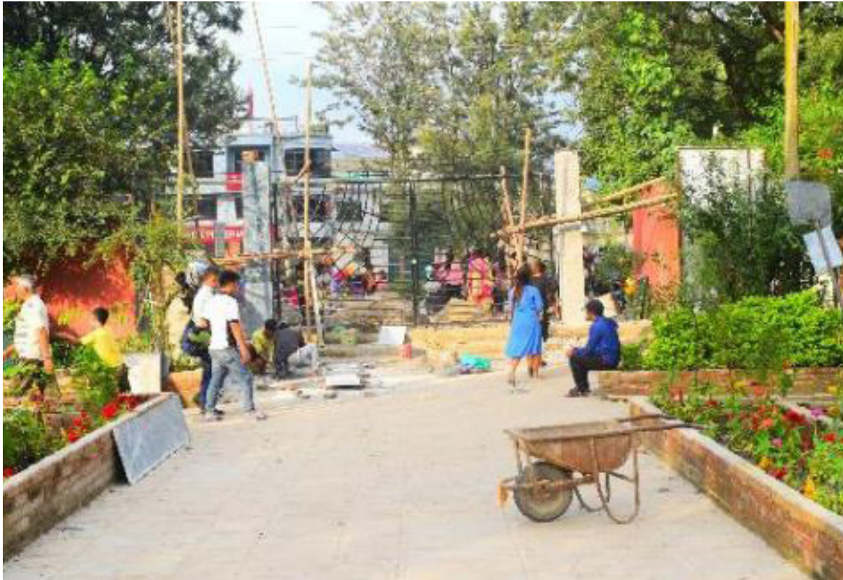
Figure 138. A gate under construction in Shankha Park
