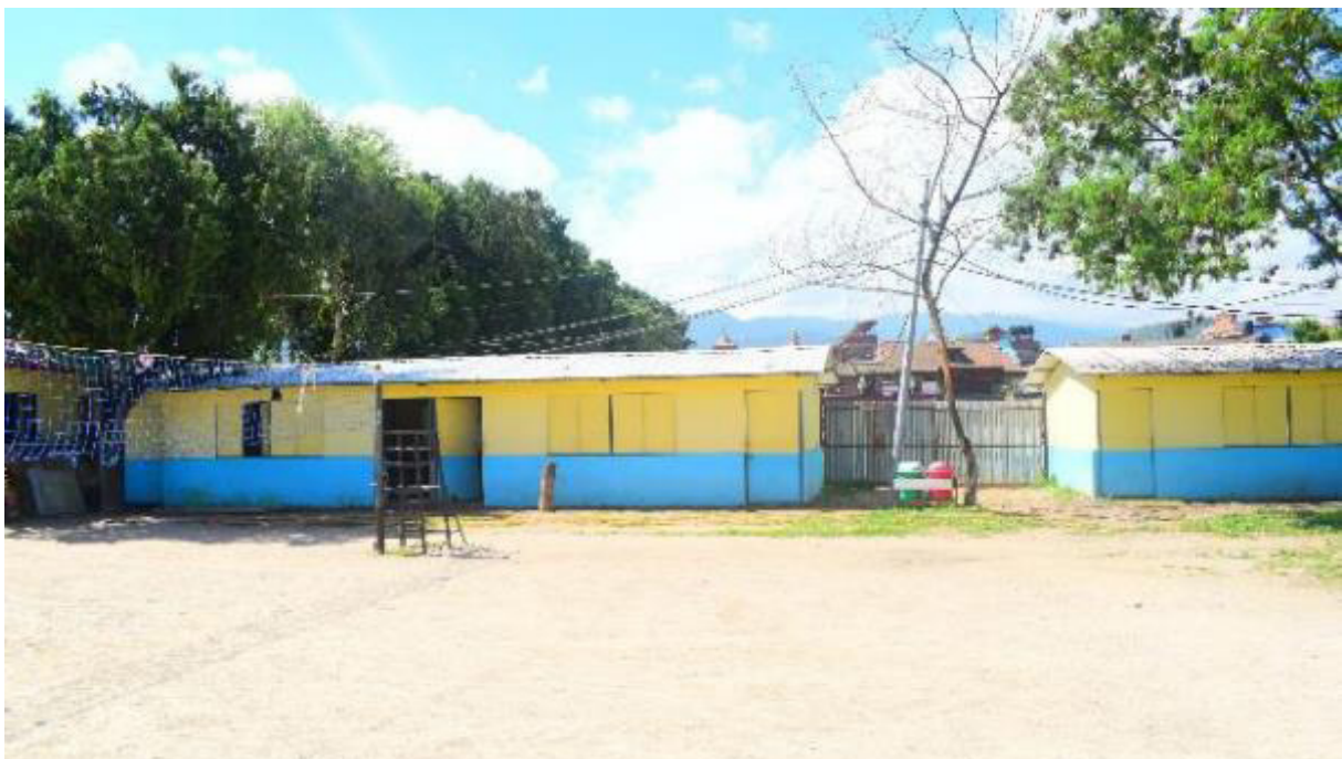
Figure 97. Newly constructed buildings in the school area
