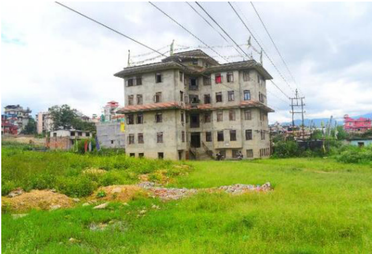
Figure 153. A newly constructed building in the Tibetan Refugee Camp
