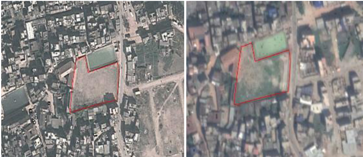
Figure 136. Aerial view of Saraswati Vidyagriha in 2013 and 2019
