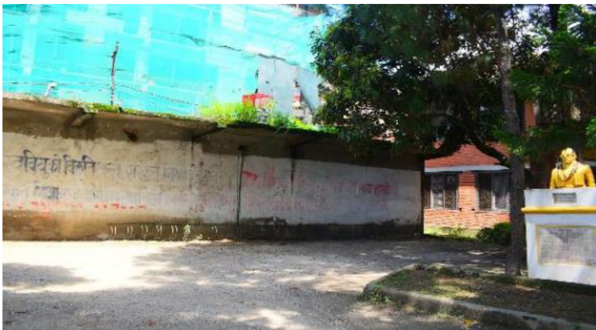
Figure 30. Construction area at Balmiki Vidyapith School premises
