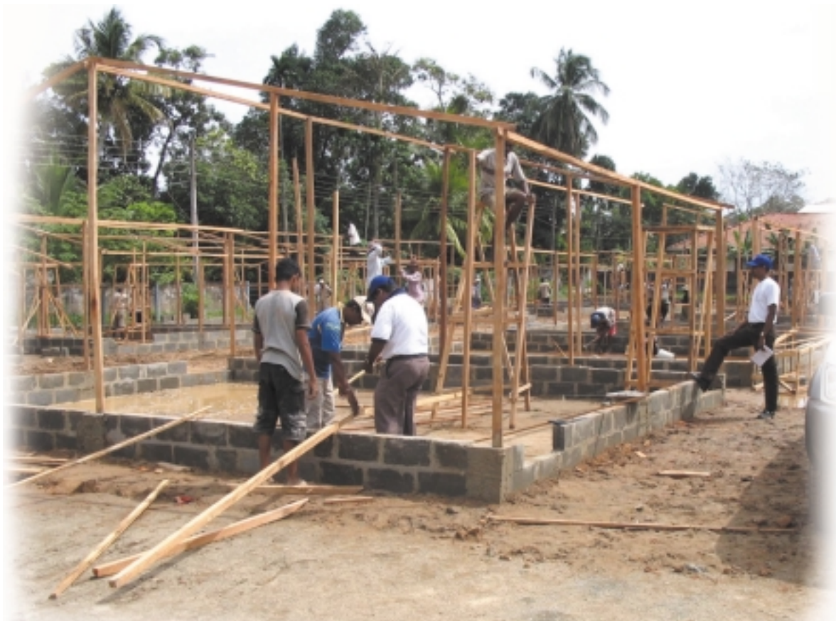
Building IOM emergency shelters in Matara Community College.
