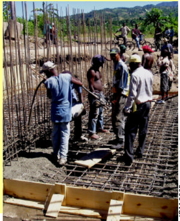
Reconstruction of the Caiman River Bridge.
