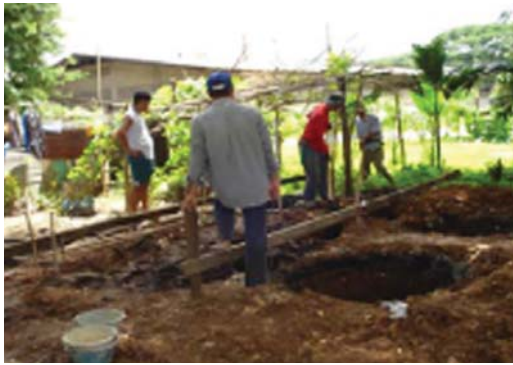
Thais and migrants in the target community build toilets with equipment and materials supported by the MHP.
