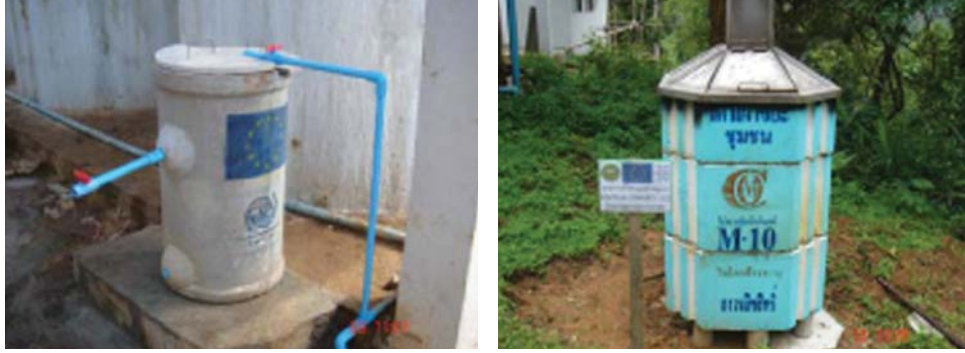
Examples of a slow-sand water filter (left) and a community incinerator (right)
