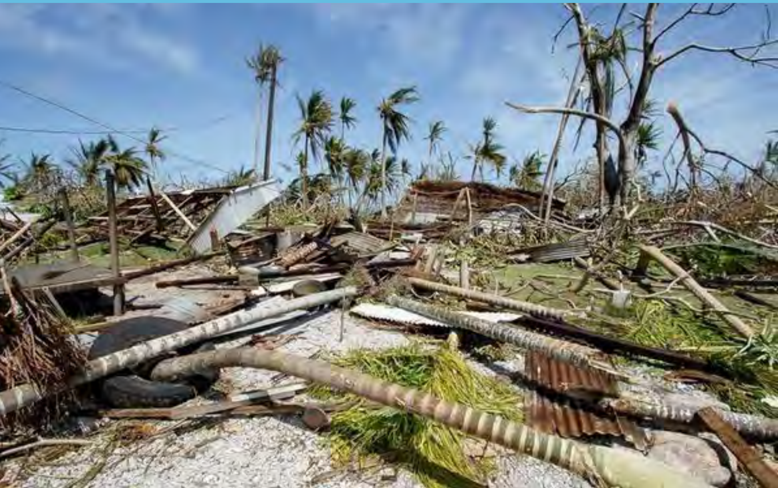
Damage caused by typhoon Maysak in Ulithi atoll in 2015. © (Photo: Brad Holland)
