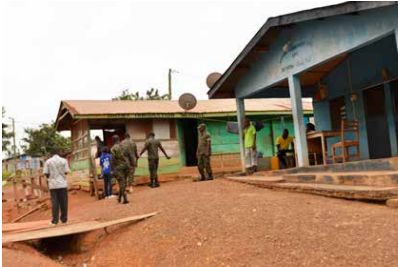
Exterior of the Antokrom BCP building. © IOM 2015
