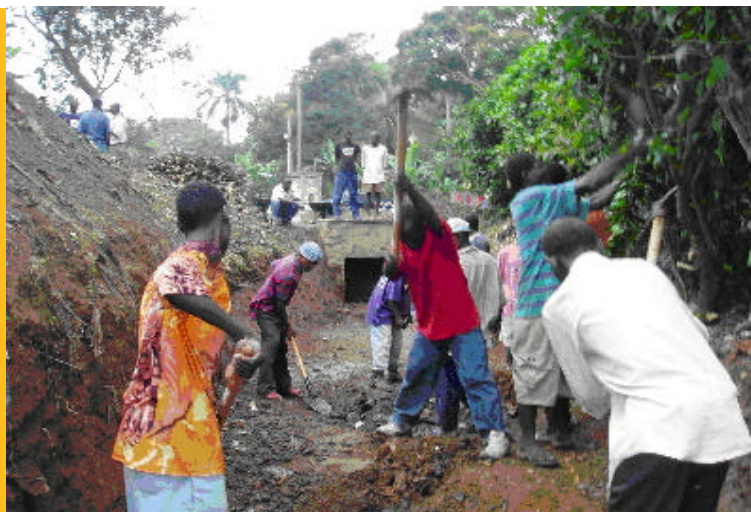
Workers in the process of transforming the canal.
