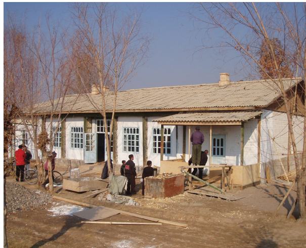
Building a community centre with pooled remittances in Tajikistan
